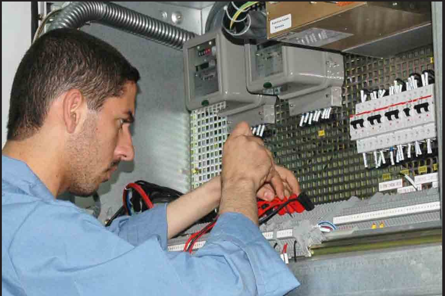
Two new 33kV substations are being constructed in Fallujah as the city's entire network is being upgraded.
