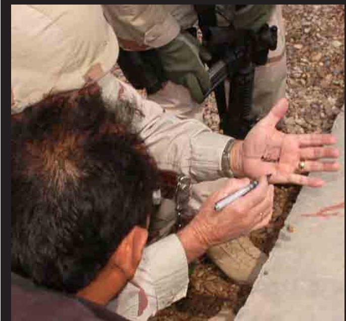
Andy May sketches out the requirements of the fuel containment area for the school's generator pad.
