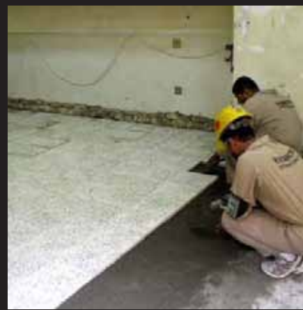
New flooring is installed.
