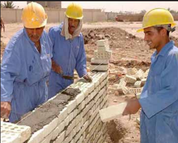
New Rusafa Courthouse taking shape in Baghdad.
