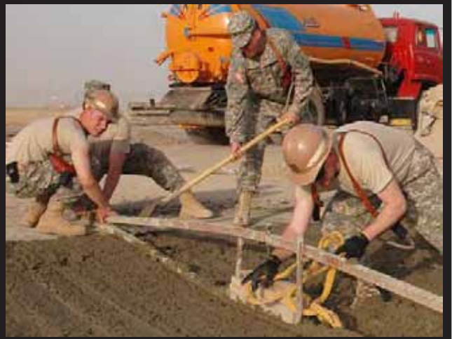
Team effort to screed the concrete.
