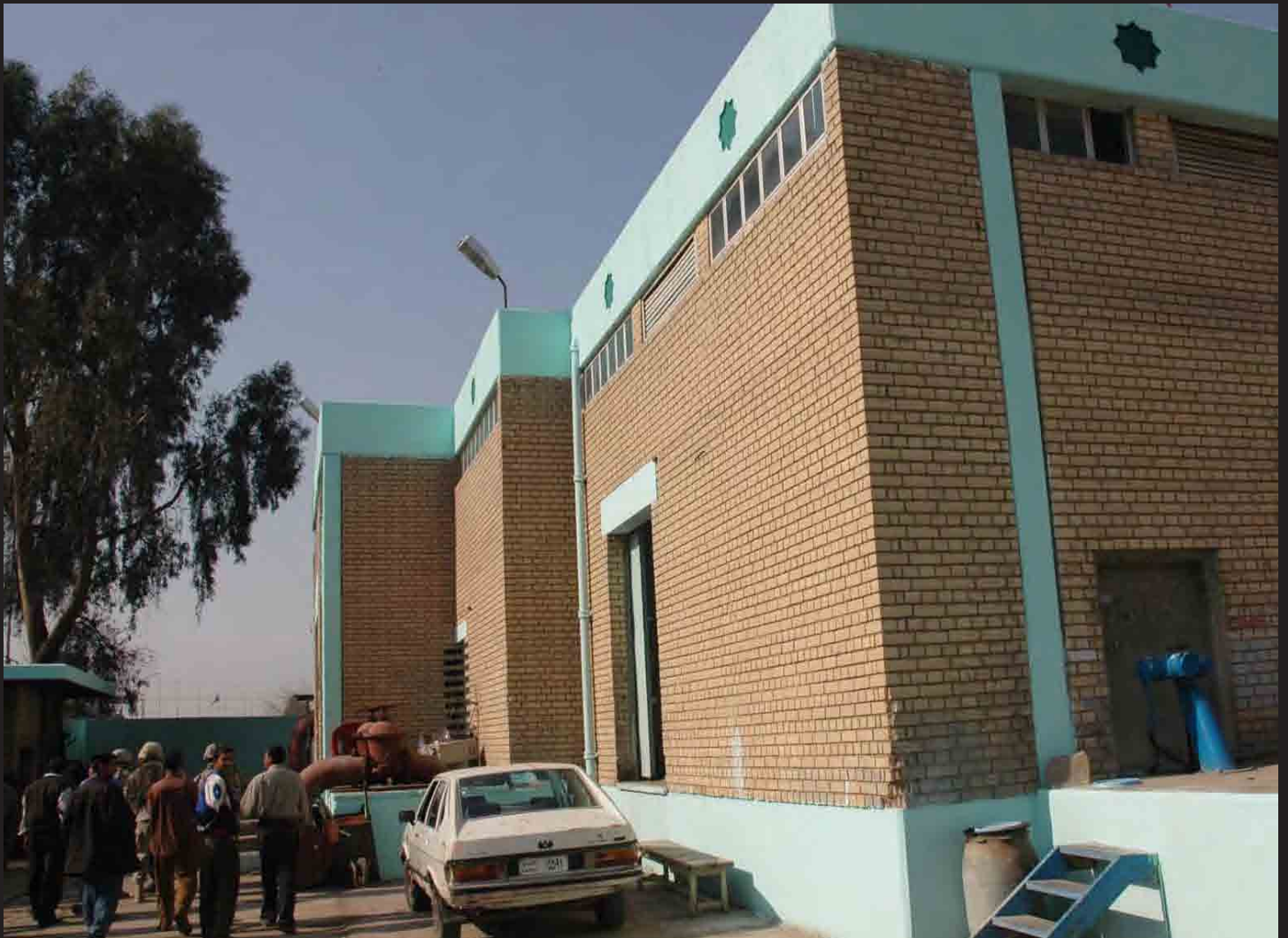
Kadamiyah Sewage Lift Station
