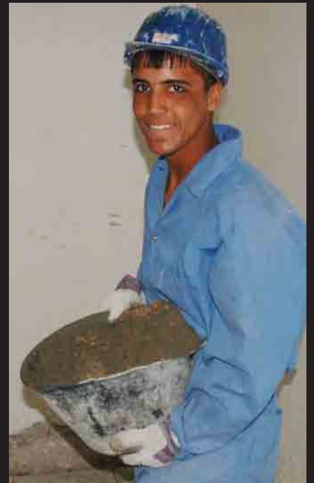
Nearly 100 Iraqi workers are helping renovate the hospital.
