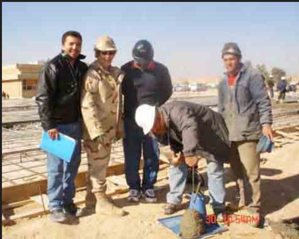
QA Rep Dorothy Ivey views concrete slump test.
