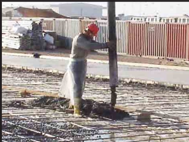
Concrete overhead from pump truck
