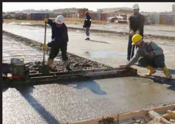
Smoothing placed concrete
