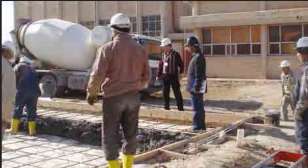
Concrete being placed
