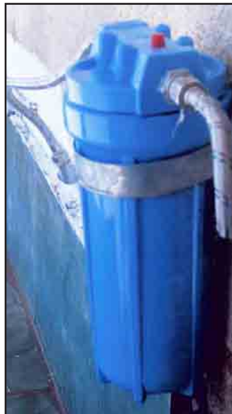
Water purification unit installed at school in Baghdad.
