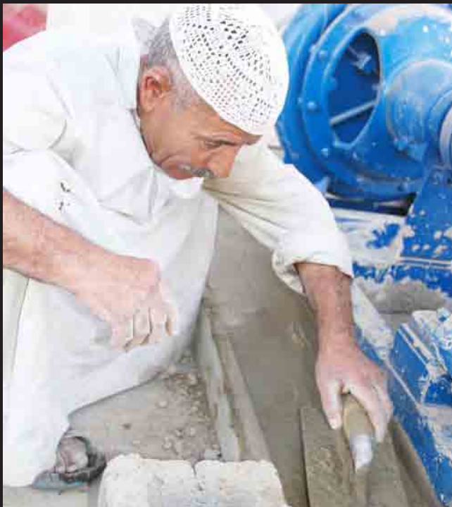
Work continues on the Al Askari water treatment plant
