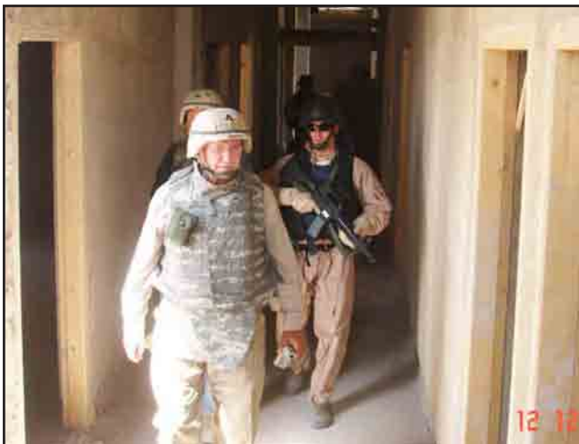
Jim Ruyak checks construction progress at Rawah Primary School, Al Anbar Province.
