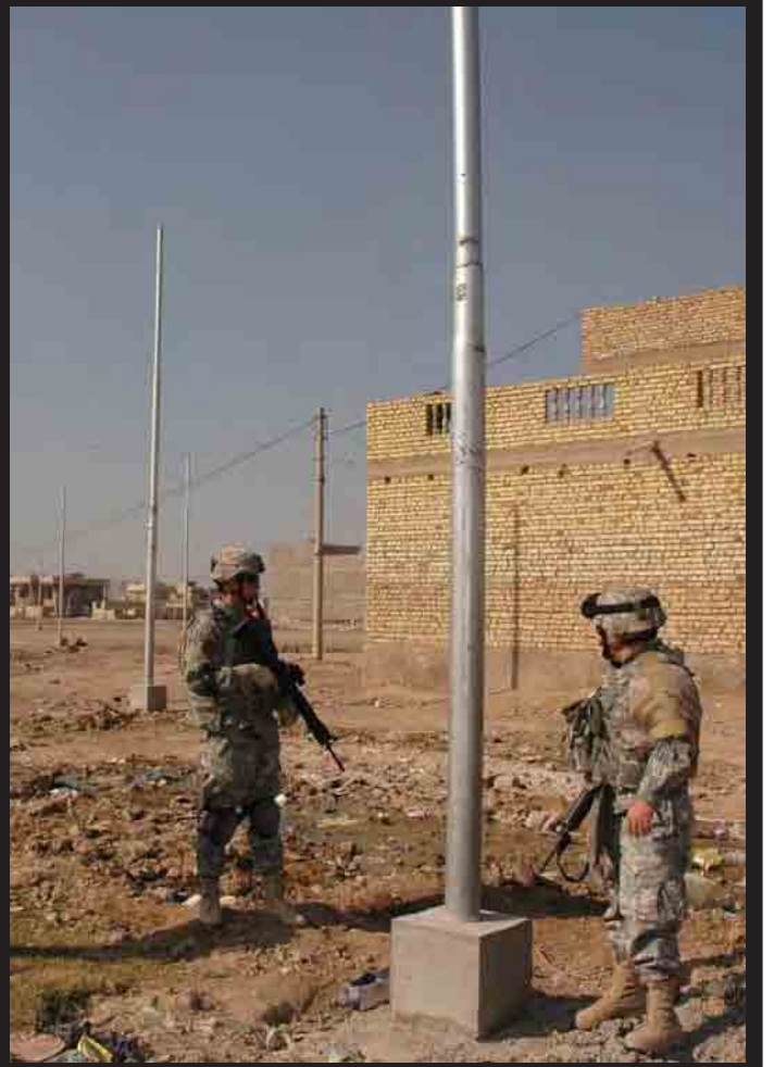
New utility poles are erected in Ghazaliya.
