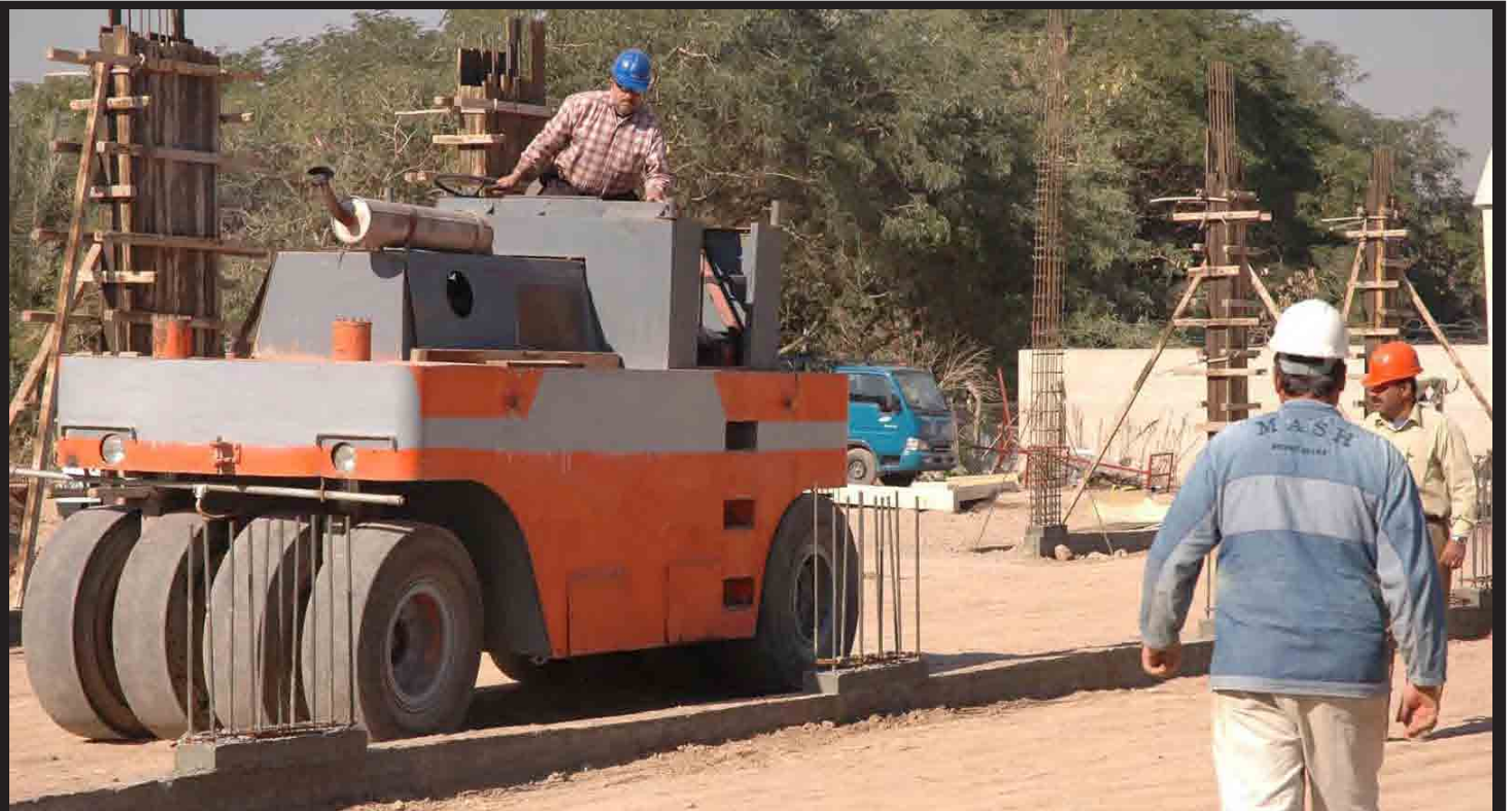
Baghdad's new Secure Documents Storage Facility now under construction
