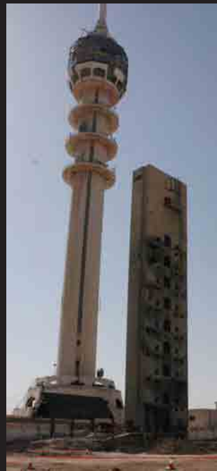
Photo at Al Mamoon before demolition
