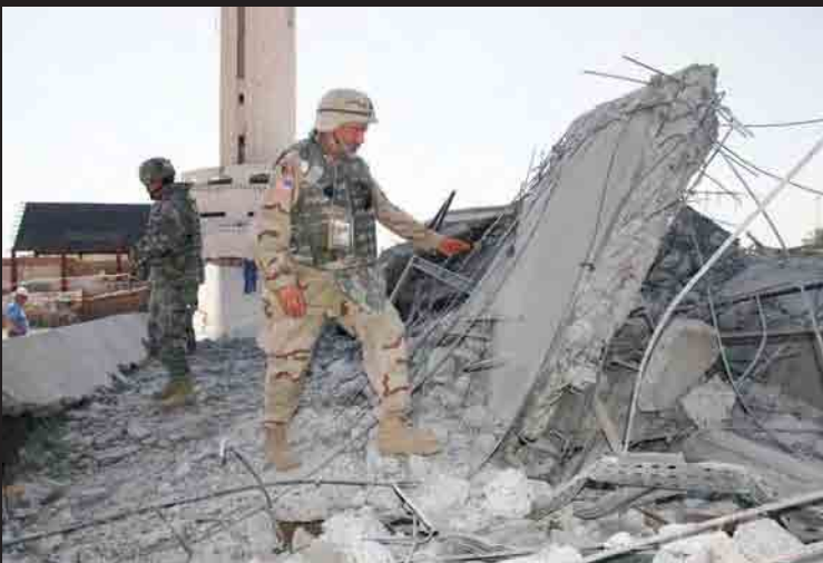
GRC IZ Office Resident Engineer Stanley Reese looks at the rubble after the 13-story concrete stairwell was flattened.
