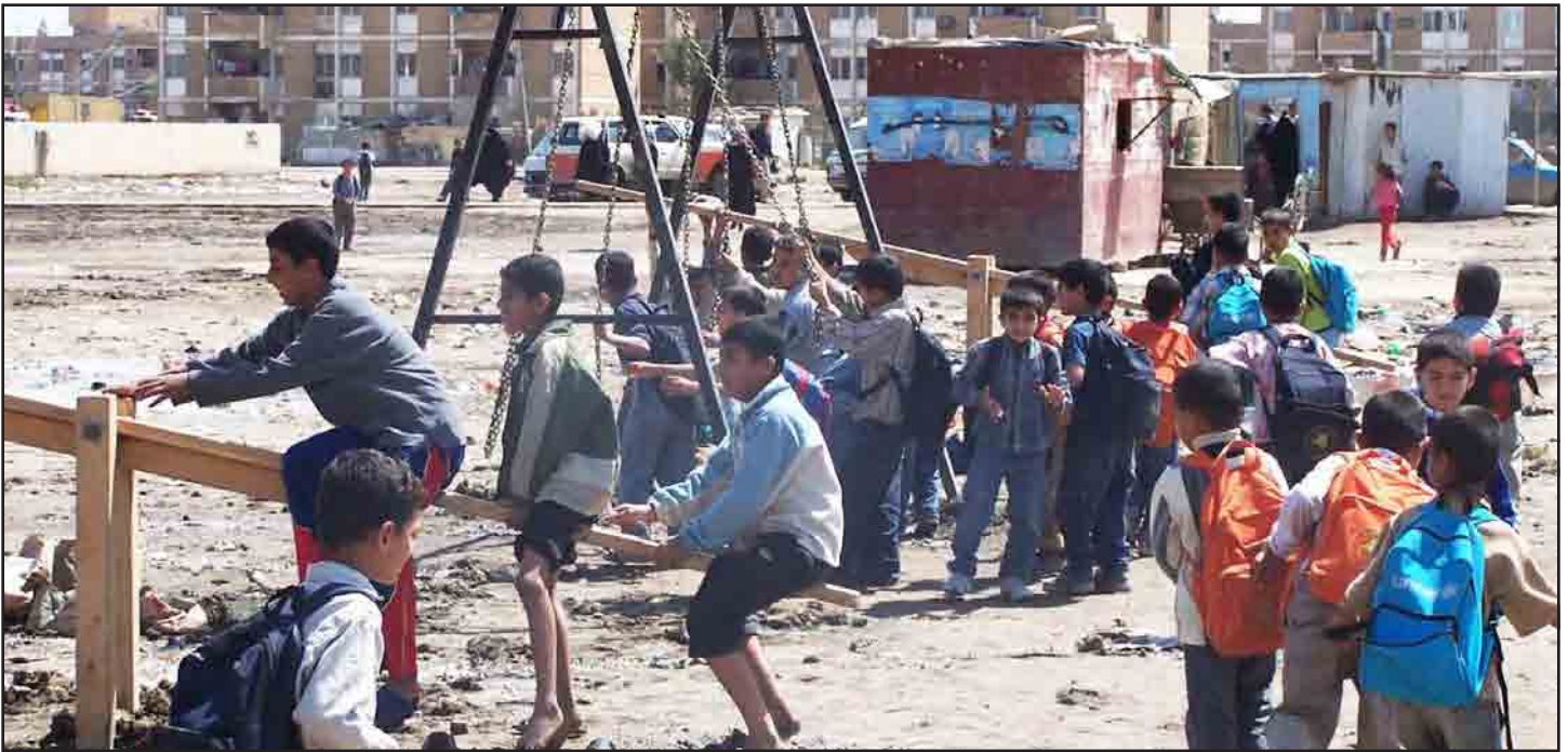
New playground equipment installed at an apartment complex in Mahmudiyah.
